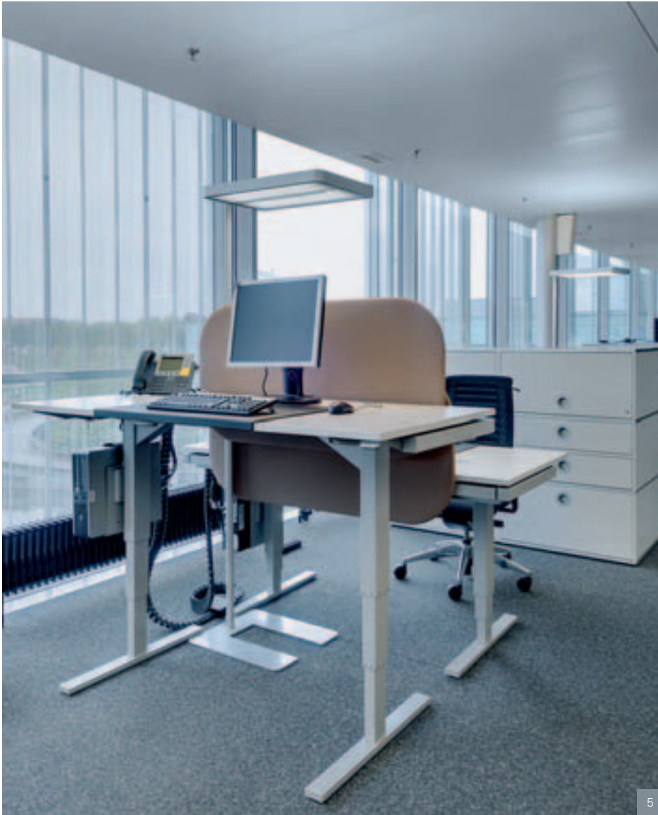
5 The free-standing luminaires automatically adjust their luminous power to the natural lighting conditions. This ensures high energy efficiency and pleasant lighting comfort.
